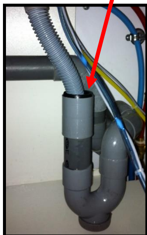
Raccordement CONFORME
