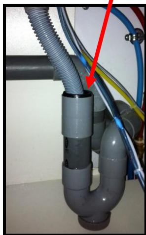
Raccordement CONFORME
