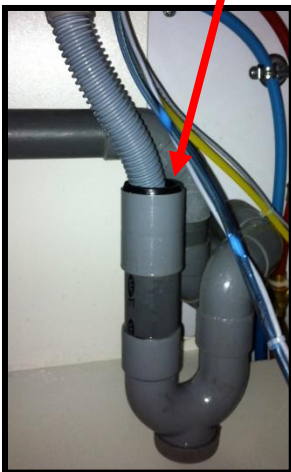
Raccordement CONFORME
